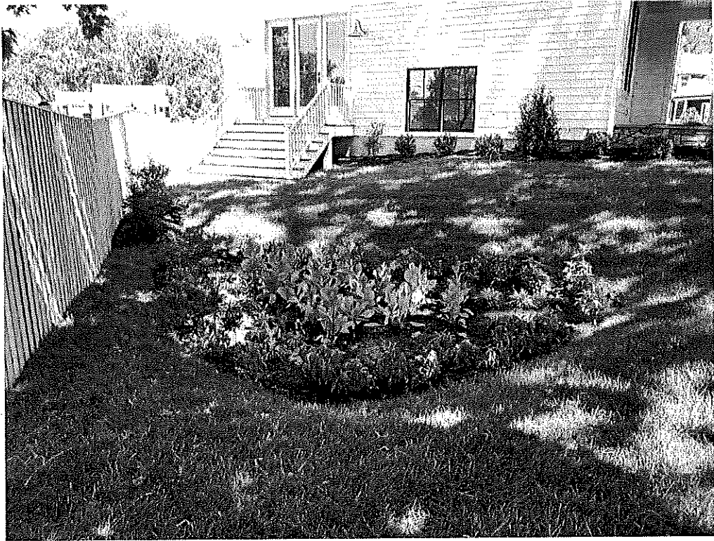
The landscape infiltration facility finished and planted.
