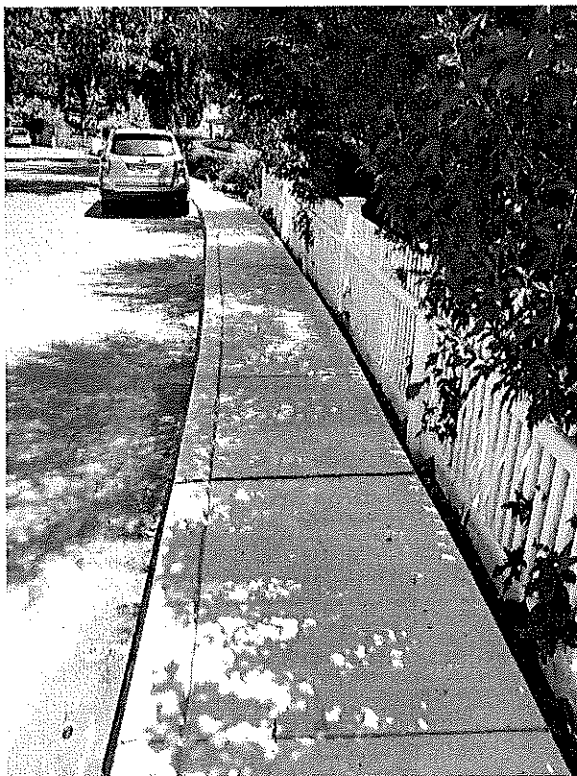
# 26 Wellesley Circle New sidewalk with a six inch high curb.
