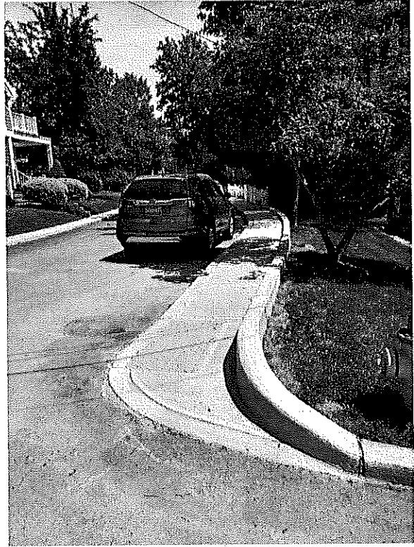
#30 Wellesley Circle with six inch high curb, and 4 inch high header curb, and detectable surface at ramp
